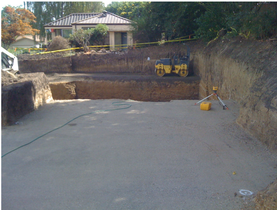
2480 Olive St. - Site side soil profile and basement excavation
