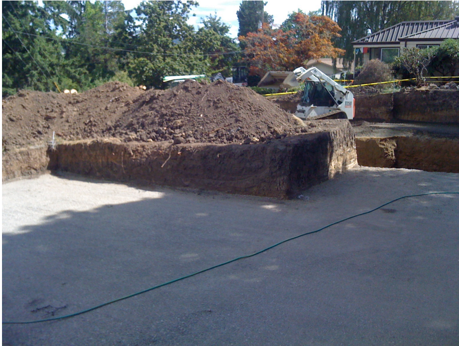
2480 Olive St. - 4" of compacted gravel on bedrock for footings
